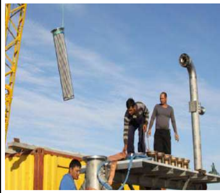
PEM 12"Flow Straightener Installion
