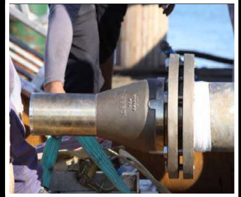
PEM 876 C being installed
