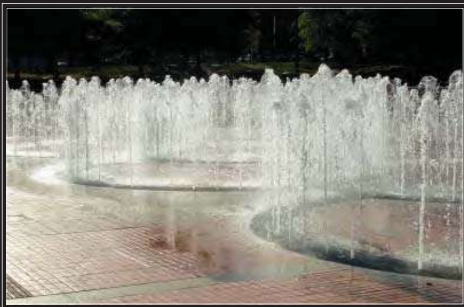
28 - 2 126 x PEM 812-2 STREAM JETS on PEM W 115-1 Water Switches & 125 x PEM 952 AERATED JETS on PEM W 115-1 Water Switches & 251 x PEM C133-8 4 COLOUR SUBMERSIBLE LIGHTS
