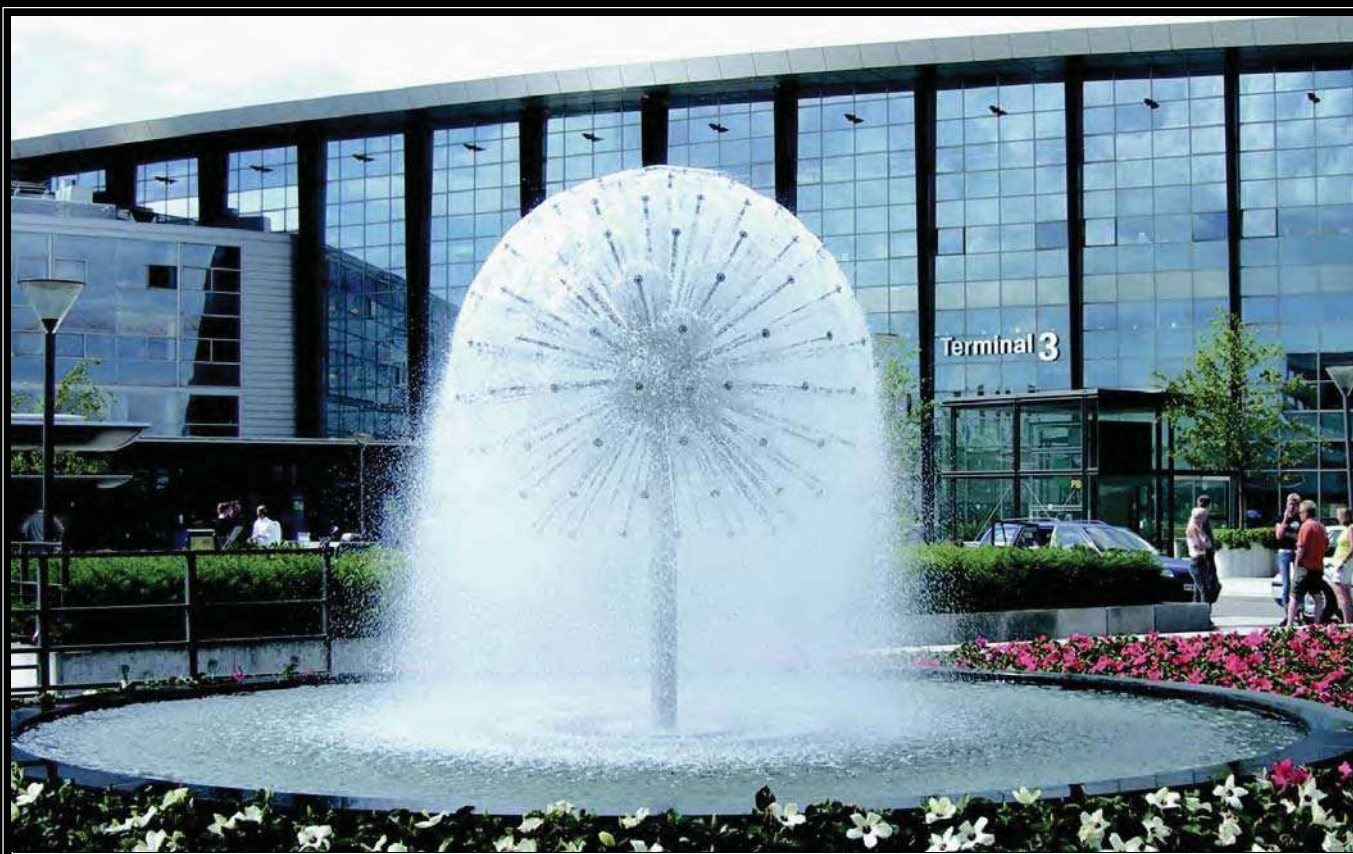
# 23 - 1 PEM 1140 at Copenhagen Airport, Denmark
